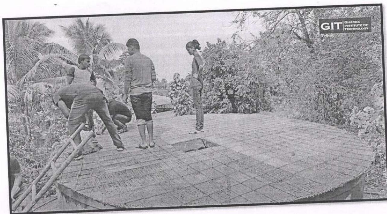
Casting of Slab of Ferrocement Water Storage Tank
